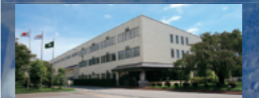
IBUKI FACTORY ▪ Vertical water-cooled diesel engine manufacturing ▪ Transmission manufacturing
