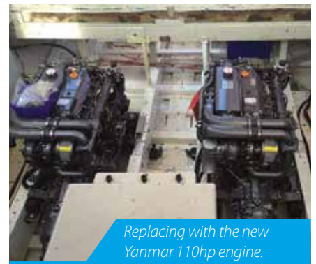
Removing the old engines.
